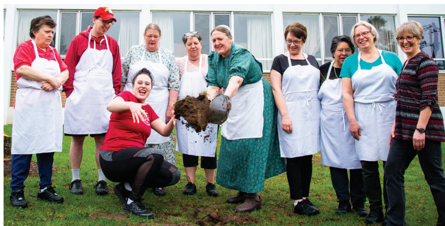
Gebel Food Services staff took their turn with the shovel in anticipation of the kitchen expansion and dining room renovation.
