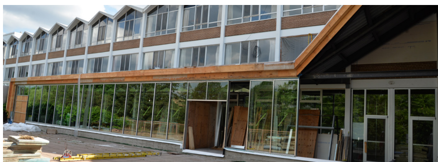
The dining room continues its transformation, as it is pushed deeper onto the patio.
